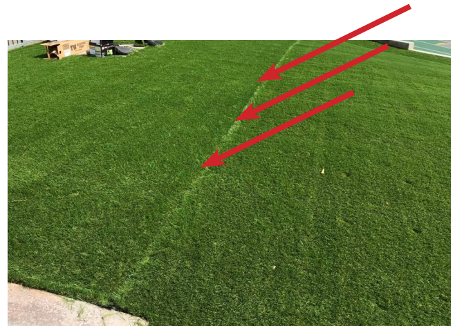
Avoid visible seams by allowing turf to stretch.
